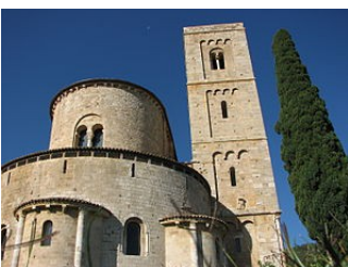
The church apse and campanile
