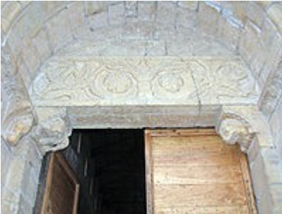
The sculpted architrave above the portal
